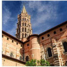
The new ZPA environmental zone of Toulouse
