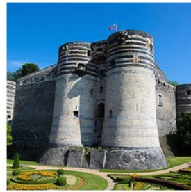
The new environmental zone ZPA of Maine-et-Loire
